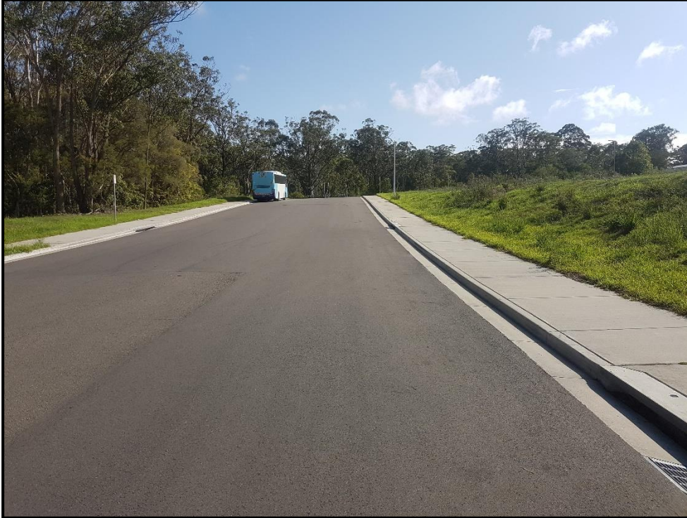
Photo 1 – Cross section of Peppertree Road looking north, subject site to the right
